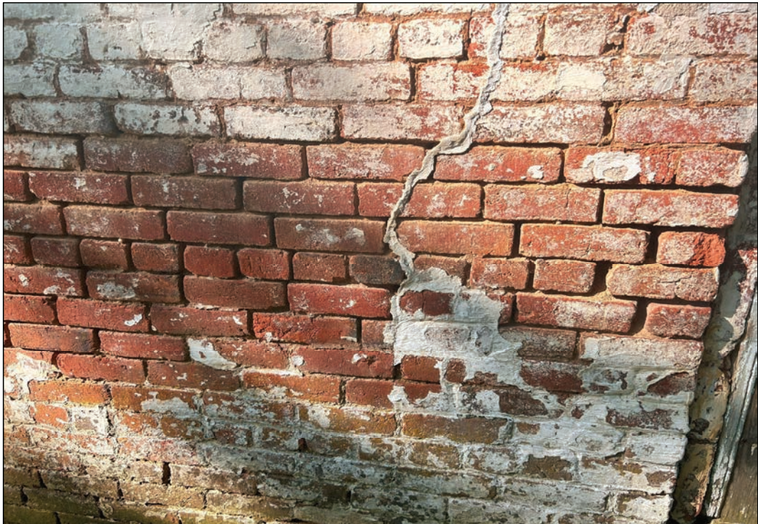
Figure 37. Northeast Elevation Common Bond Brick Wall. Note Deteriorated limewash and mortar failure. -
